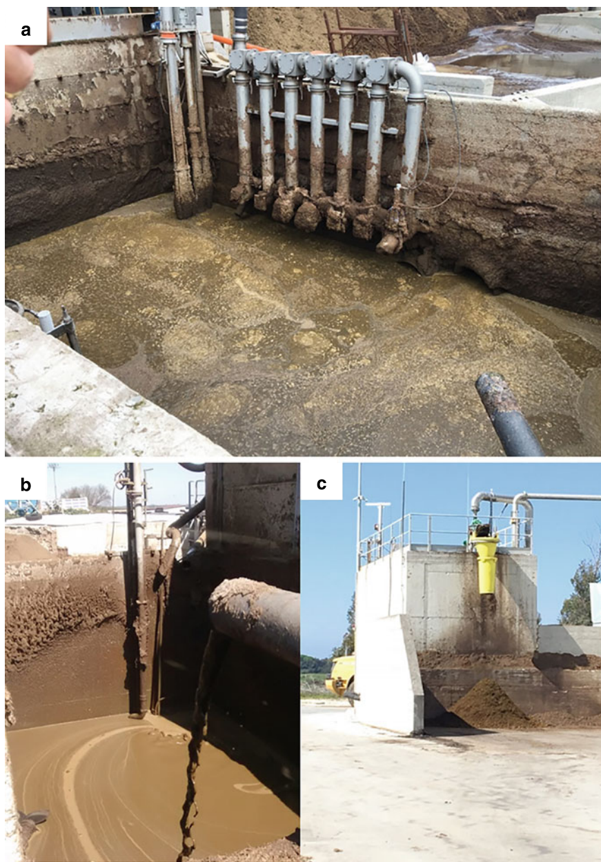
Fig. 3 Pictures of an open-air tank where manure is stored before entering the digester (a), exit pipe of digestate after the digestion process (b) and storage of solid digestate after solid/liquid separation process (c)
