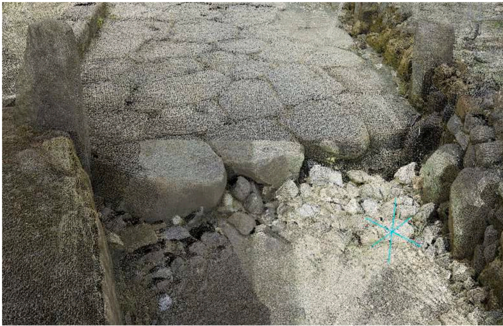
Fig. 4. Point cloud representation in Leica Cyclone of the step between the un-paved and the paved road stretch.
