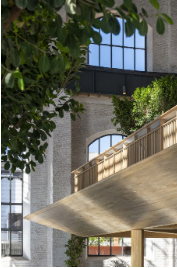
Fig. 10. Interior view of building. The historic building envelope has been retained to conserve over 10,000 tonnes of original brick and mitigate the environmental impact. The lightweight structure inserted inside the space is made from sustainably sourced timber from local forests and allows for spatial flexibility (image: © Nigel Young / Foster+Partners).
