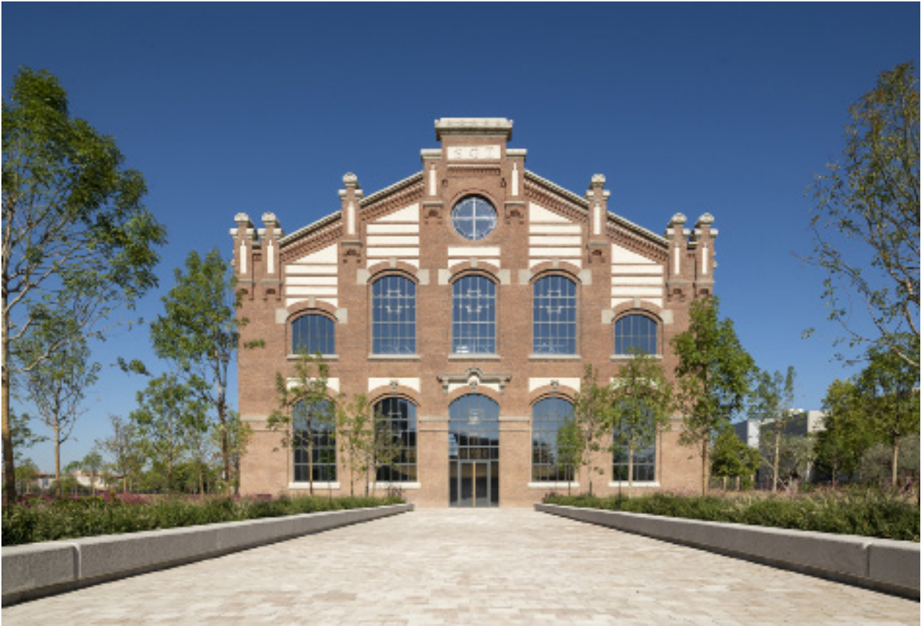
Fig. 1. Exterior view of building. Originally built in 1905 by the architect Luis de Landeche, the building once supplied energy to the surrounding areas. It later fell into disuse until ACCIONA acquired it in 2017, saving it from demolition, a fate that other similar structures in the area had experienced in recent years (image: © Nigel Young / Foster+Partners).
