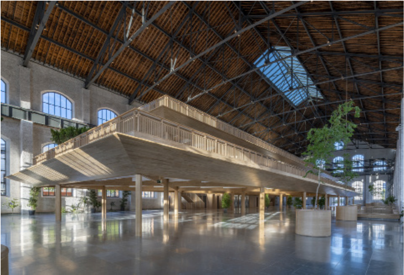
Fig. 3. The lightweight structure inserted inside the space is made from sustainably sourced timber from local forests and allows for spatial flexibility (image: © Nigel Young / Foster+Partners).
