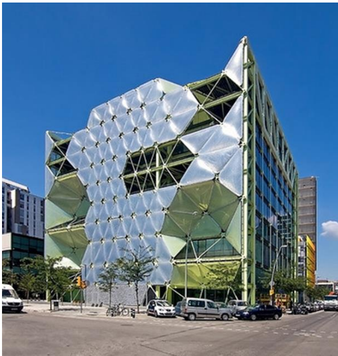
Fig. 5 - MEDIA-ICT BUILDING BARCELONA (Barcelona Growth Center ): example of a smart-eco-self-sufficient building
