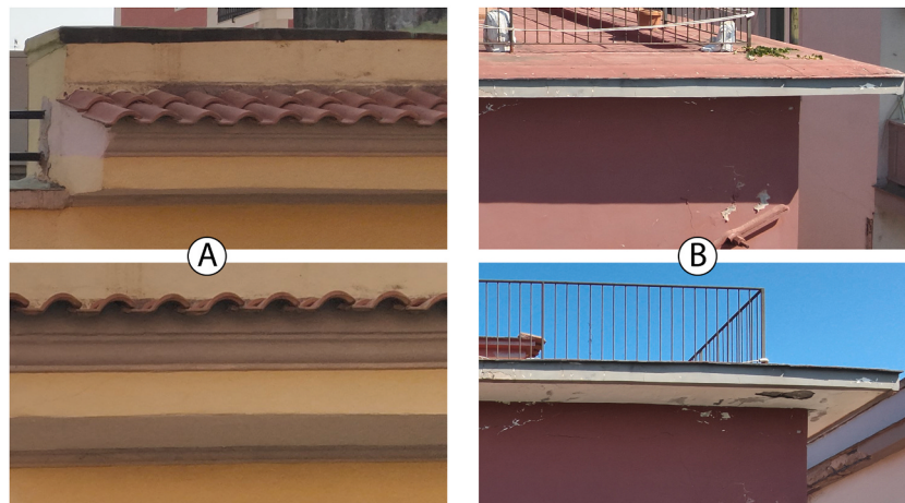
Fig. 3. – Examples of a masonry roof cornice (Fig. 3a, left) and a reinforced concrete roof cornice (Fig. 3b, right).
