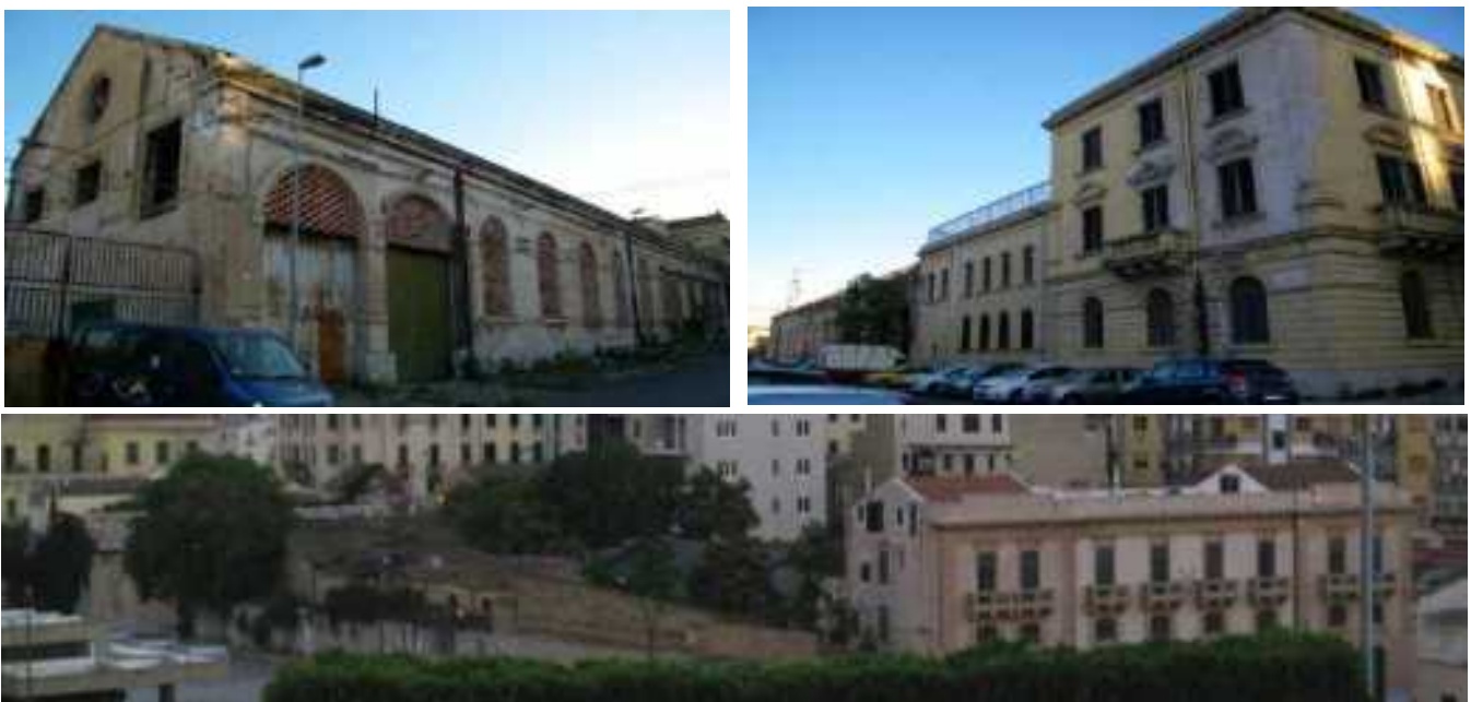
Figure 5. (a), (b) The power station at coal. (c) Residential buildings.
