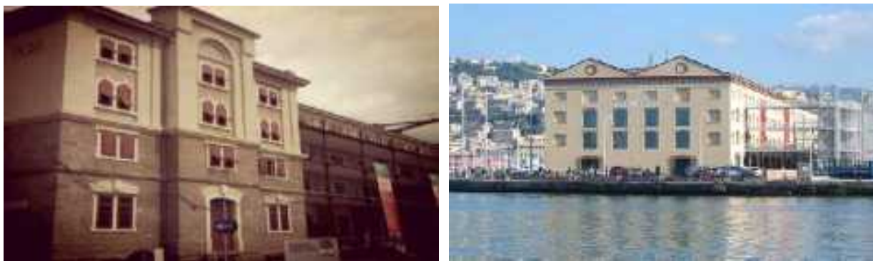
Figure 7. (a) Trieste: the warehouse 26. (b) Genova: the former cotton warehouses.
