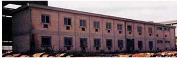
Figure 1. The building tested within the ILVA-IDEM research project before experimentation.
