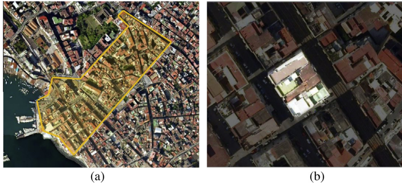
Fig. 25. The investigation pilot area (a) and the bird-eye view of the study masonry aggregate (b) of the historical centre of Torre del Greco.
