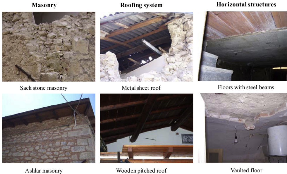
Fig. 37. Main structural features of masonry aggregates of Poggio Picenze.
