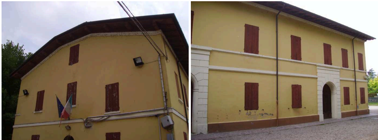
Fig. 3. The main facades of the school building "Sorelle Luppi"
