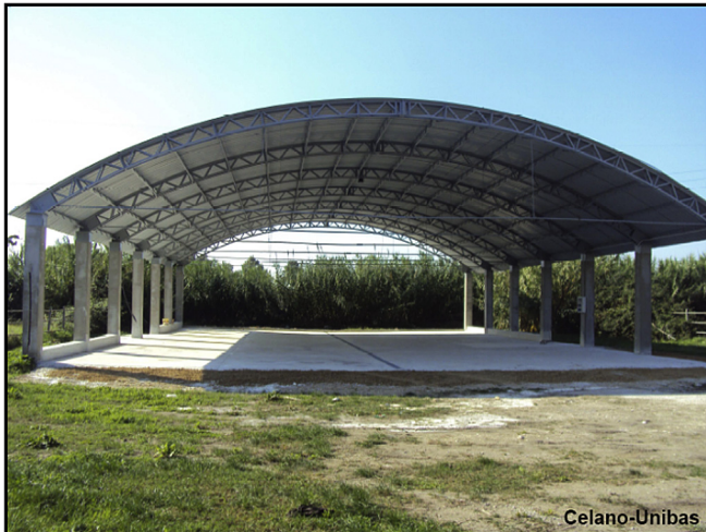
Fig. 1. Castel Volturno composting plant (CV Plant).
