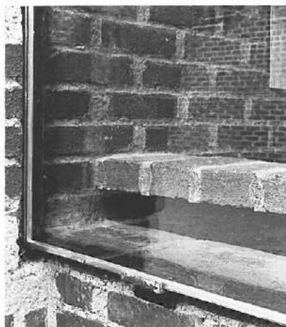
Building details of the door and window frames.
