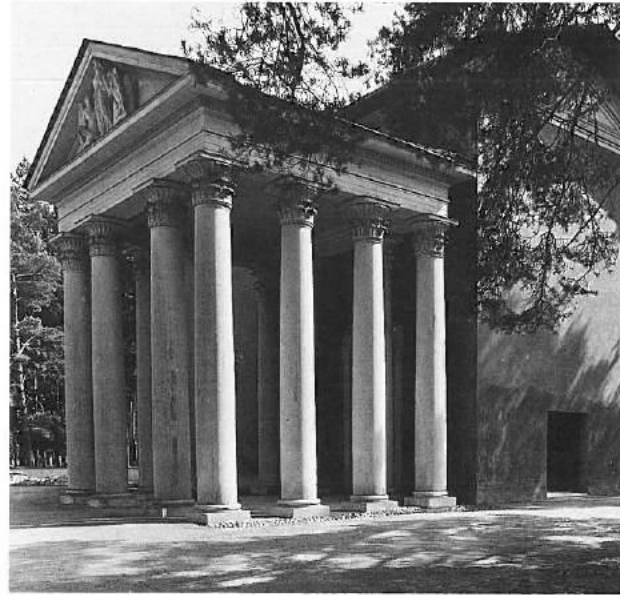
Entrance portico and the access road.
