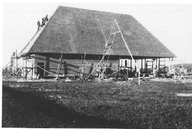
Kvarnsveden Cemetery, the funerary chapel under construction.
