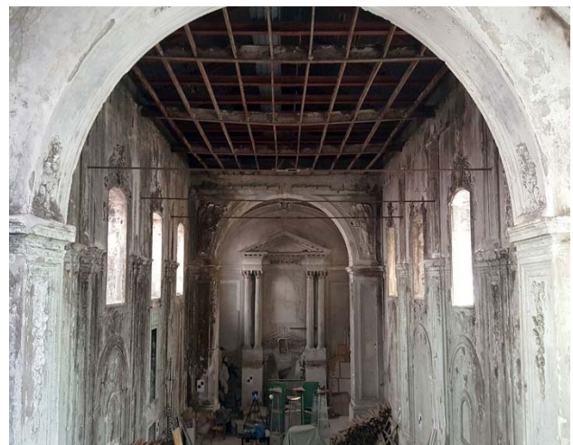
Figure 1: Indoor view of the Church of Rosario di Palazzo.
