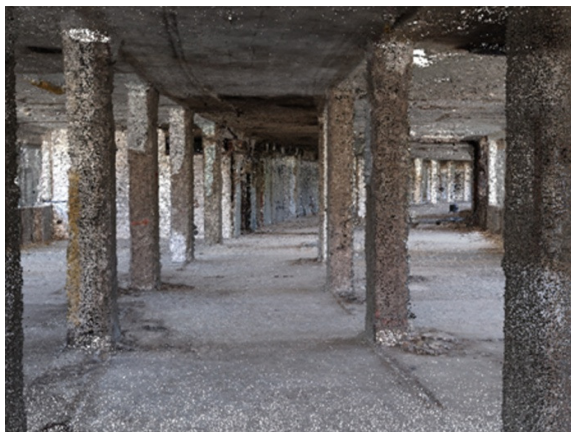
Figure 4: Internal view of a point cloud of a standard level.
