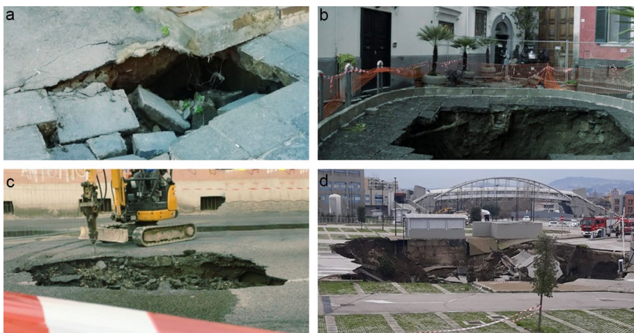
Fig. 3 Examples of sinkholes located in the city of Naples: a Via Girolamo Santacroce, Vomero municipality, 15/02/2019; b viale Calascione a Monte di Dio, 08/11/2019; c via Jacopo De Gennaro, Fuorigrotta municipality, 18/12/2019 (modified from www.ilmattino.it ); d parking of Ospedale del Mare, 08/01/2021
