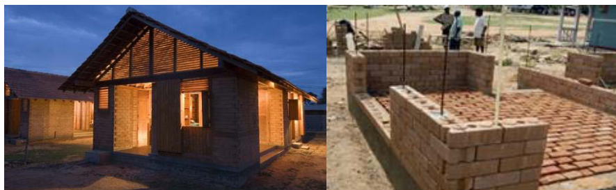
Figura 1 – Post-Tsunami Housing, Kirinda (Sri Lanka) – Legno, blocchi in terra compressa, tegole – Shigeru Ban (2006).
