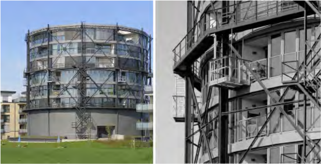
Fig. 11. Gasometer in Stade, Germany. Gerhard Buttge Architect. Housing Project, 2015 (source: Buttge Architects website).
