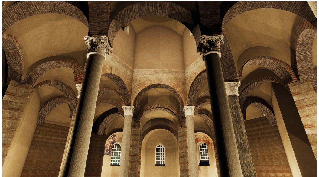
Figure 13. A rendered view of the interior of the church showing the complex structure of the vaults covering the inner and outer ambulacra. Remains of early medieval frescoes are visible on the apsidal basins [34].
