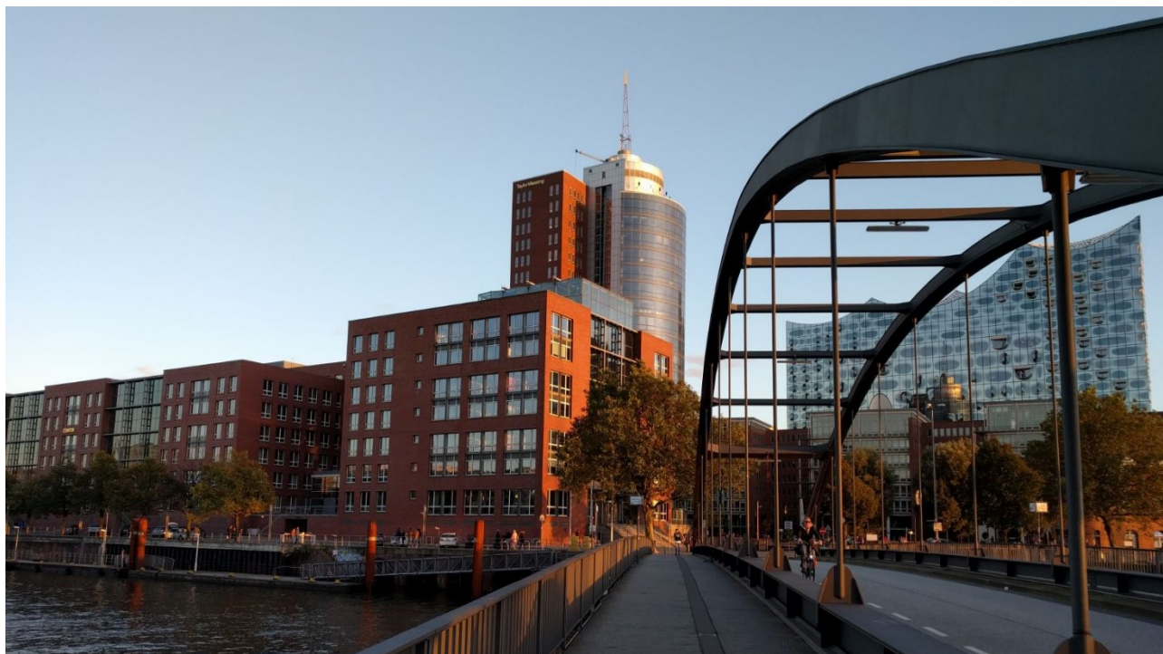
Figure 4: Hamburg, Niederbaumbrücke: the connection to Hafencity. Photo by F. Vingelli, 2017.
