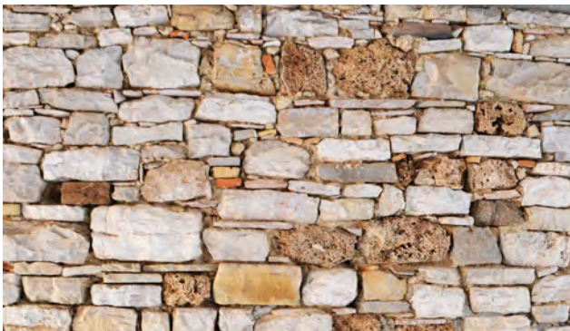
Figure 4. Frosolone (Isernia, Italy): the photo shows a masonry of limestone and cimenti (Romano, 2016).
