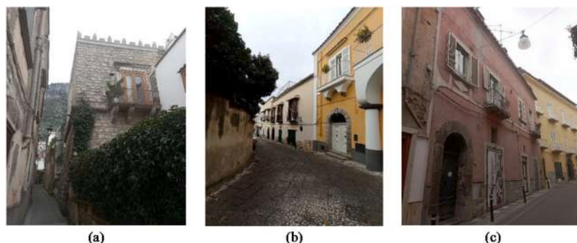
Fig. 4. Curtains of buildings along (a) Via Olivari, (b) Via Santa Lucia and (c) Via A. Cosenza.
