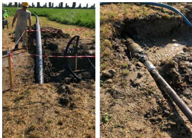
Fig. 24 Final withdrawal of HD well screens, starting point (left) final point (right)
