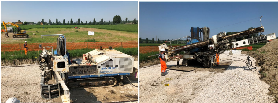
Fig. 22 Drilling equipment set-up during directional drilling activities
