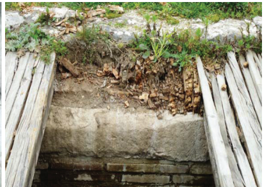
Fig. 4 – Bearing on stone elements (“B”)
