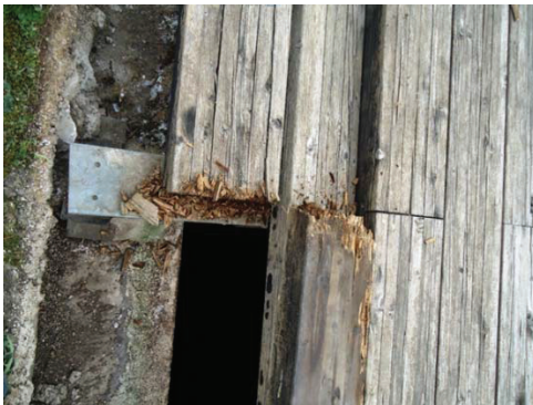
Fig. 3 – Bearing on steel profiles (“A”)
