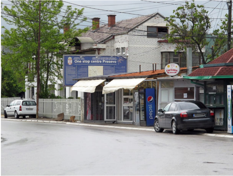
Fig. 2 One Stop Centre in Preševo, outside the camp—May 2016. Photo by the authors
