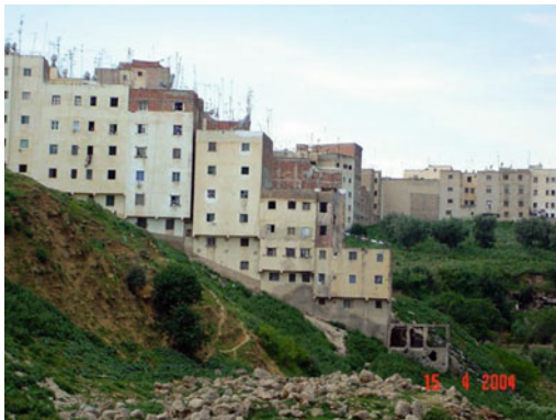
Photograph 1 Constructions in the form of staircases, backed up and raised in height, built on marly lands on steep slopes, near the stream (Oued Fès). They are threatened with collapse due to landslides on these cliffs (Northeast zone of Fez)
